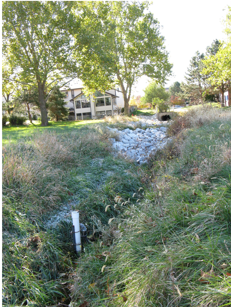
Figure 3.6: Taylor Park Monitoring Site, Facing South.
