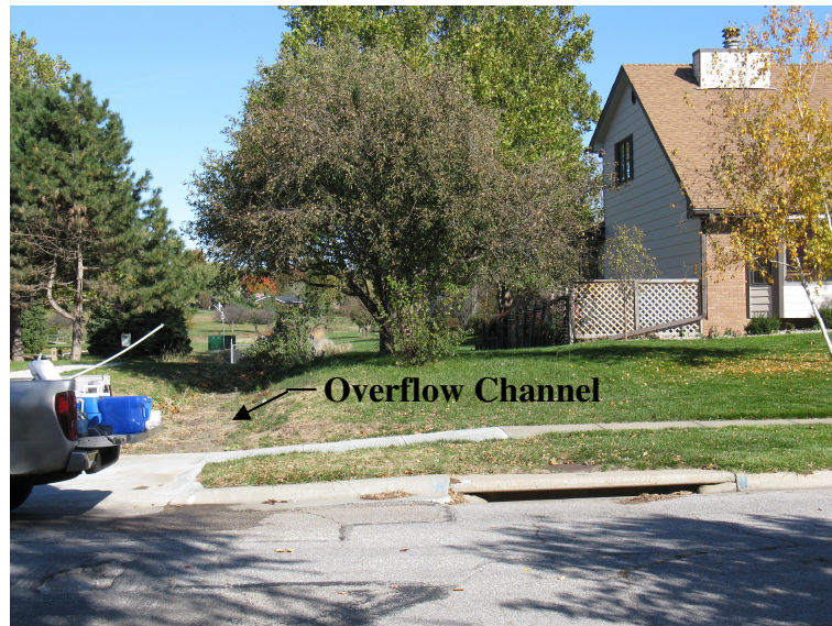
Figure 3.7: Overflow Channel at the Taylor Park Site
